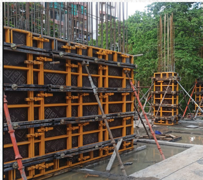
STANDARD BELEX FORM WORK SYSTEM
