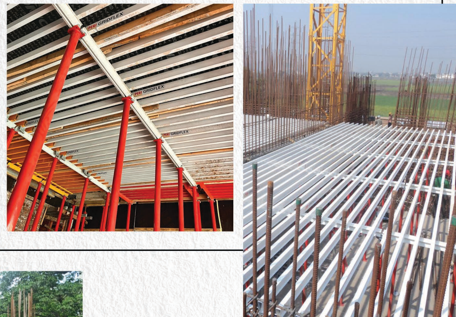
GRIDFLEX SHUTTERING FORM WORK
