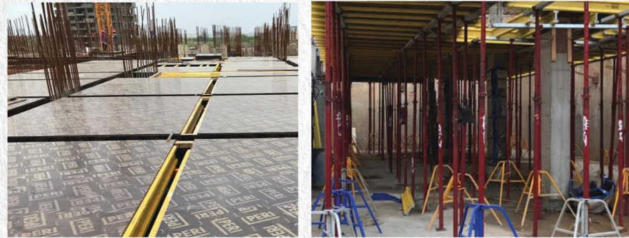
GRIDFLEX SHUTTERING FORM WORK
